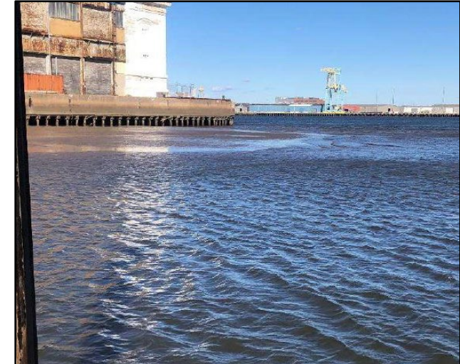
Severe shoaling of boat basin at Sector Delaware Bay
