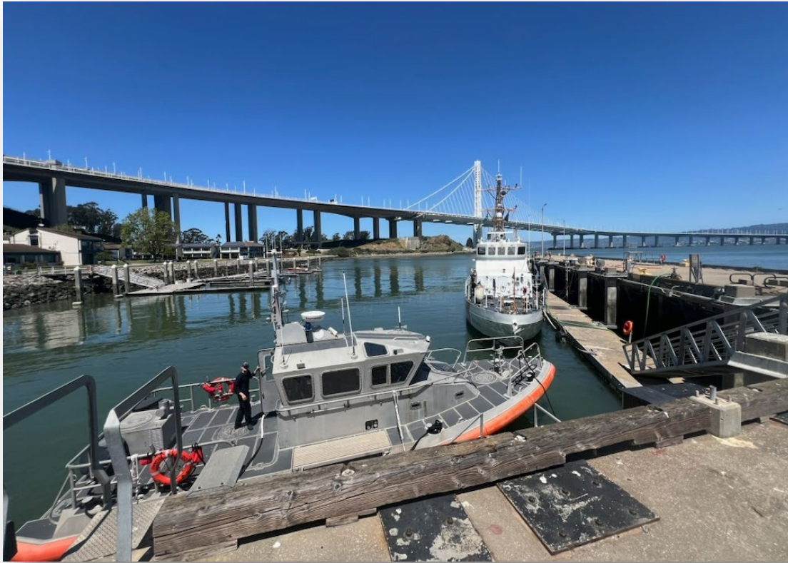
Damaged piers at Sector San Francisco, CA
